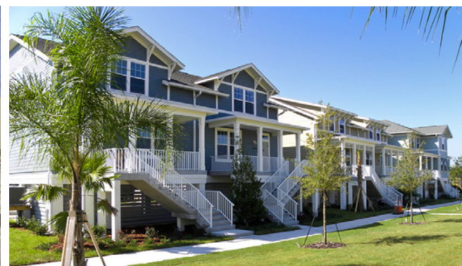
Facility Group 4 Family Housing, Facility Group 4 MacDill AFB, Florida Torti Gallas and Partners, Architect Photo Courtesy US Air Force Civil Engineer Center
