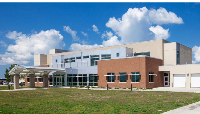
Facility Group 2 Base Operations Facility Minot AFB, North Dakota Leo A Daly, Architect Photo Courtesy US Air Force Civil Engineer Center
