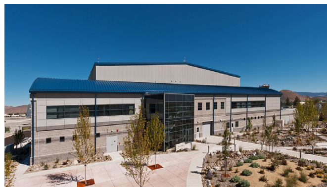
Facility Group 3 Maintenance Hangar Reno, Nevada H+K Architects Photo Courtesy US Air Force Civil Engineer Center
